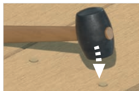
5. Press caps with a rubber mallet
